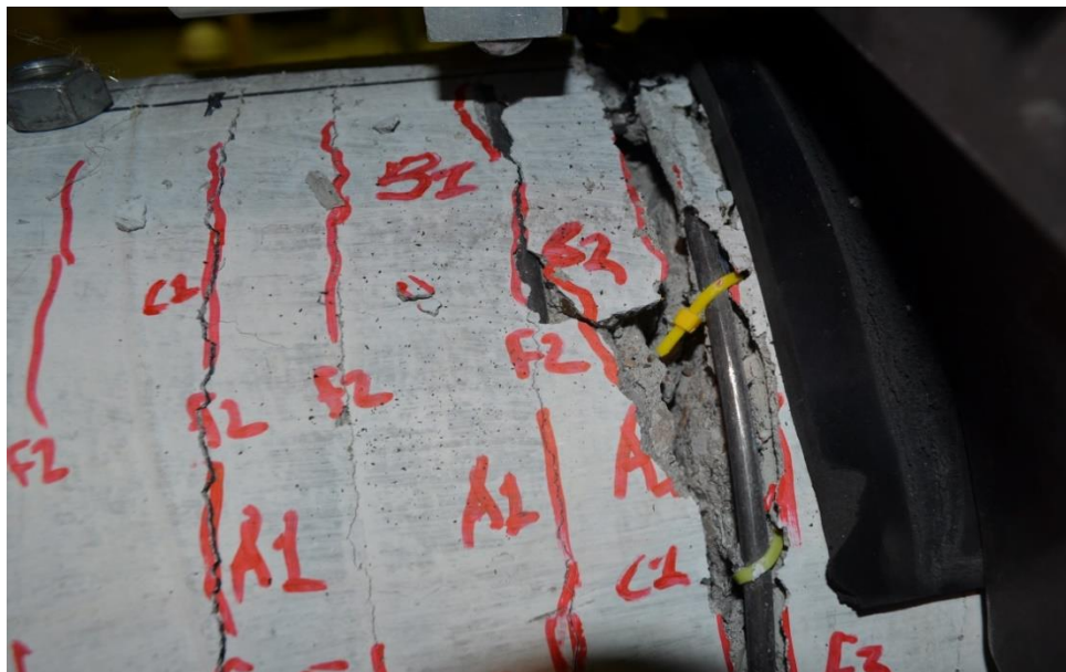
Figure 5-7: Close-Up View of Large Flexural Crack in Specimen SC2-C
