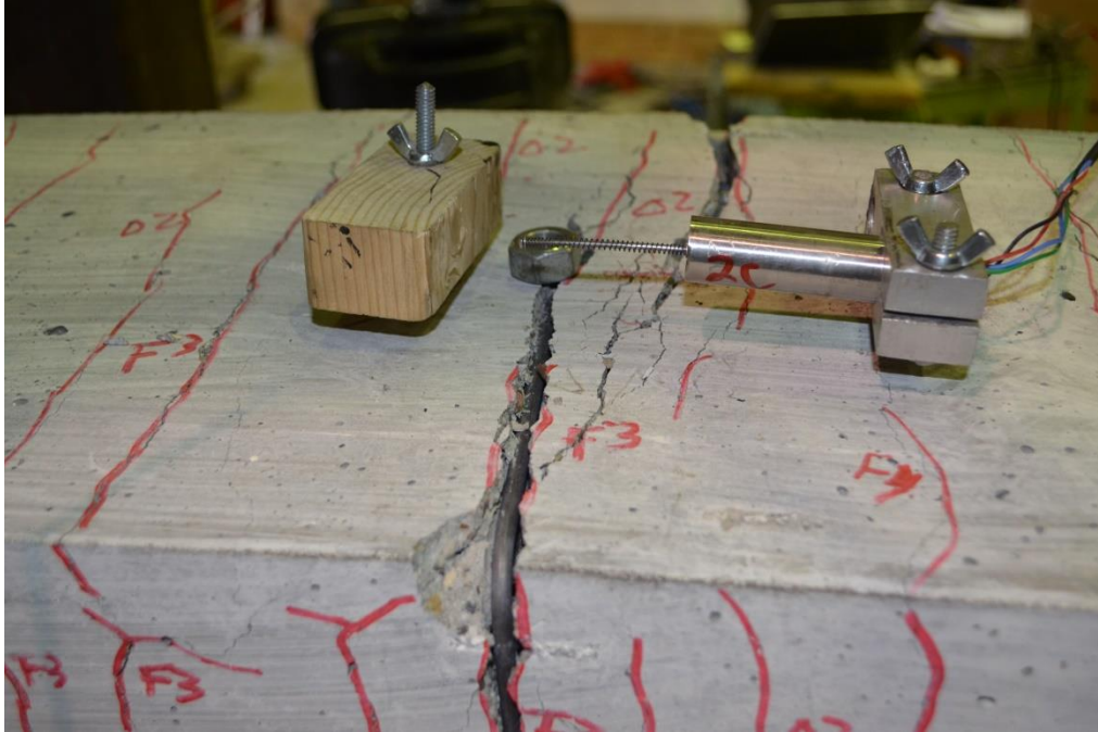
Figure 5-61: Specimen SS1-M Close-Up of Large Flexural Crack after Failure
